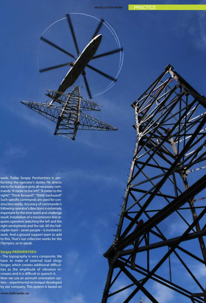
using a bilateral suspender with a two-point load fastening. The load may be stabilized and moved with on-board LPG-300 hoists. The load may be turned in azimuth in plane parallel to the main rotor plane. When the helicopter approaches an erection joint, the load is orientated in the direction convenient for alignment of technological axes. The equipment, which we use, is not in mass production.
